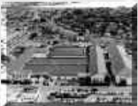
**This overhead view of the Air Force Personnel Center (AFPC) shows how builders joined two of the old enlisted barracks to form a new facility. To the right, a third building is also connected to the AFPC complex. It was built in the mid-1960s when AFPC came to Randolph AFB.**
